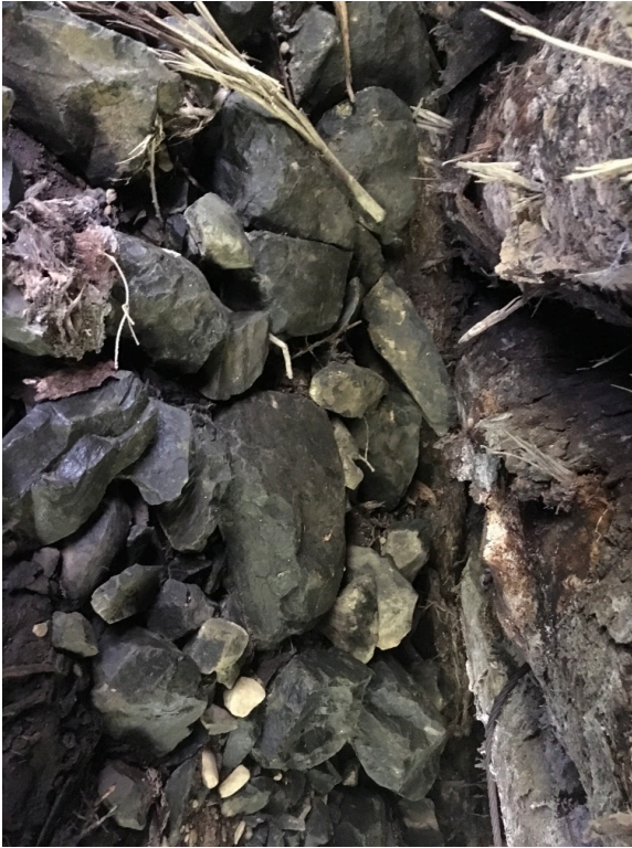
Right Bank Abutment when facing downstream
